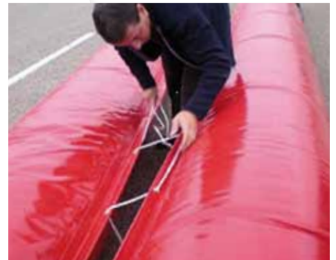
Laçage des 2 tubes Lacing the two tubes
