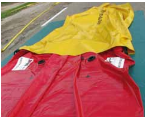
Mise en place des manchettes Establishment of the connection
